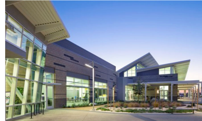
Eastvale Community Center, Eastvale
