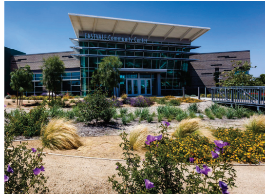
Eastvale Community Center, Eastvale
