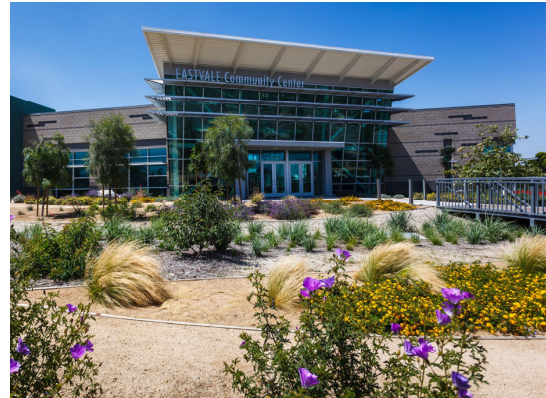
Eastvale Community Center, Eastvale
